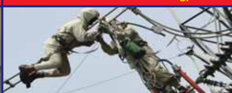
Bypass Jumper Works in 66kV Switchyard at HLTC Bangalore
