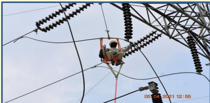
Live Line Maintenance at 400 KV
