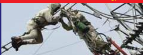
Bypass Jumper Works in 66kV Switchyard at HLTC Bangalore
